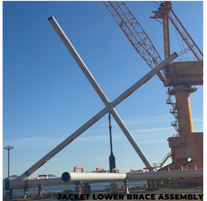
JACKET LOWER BRACE ASSEMBLY
